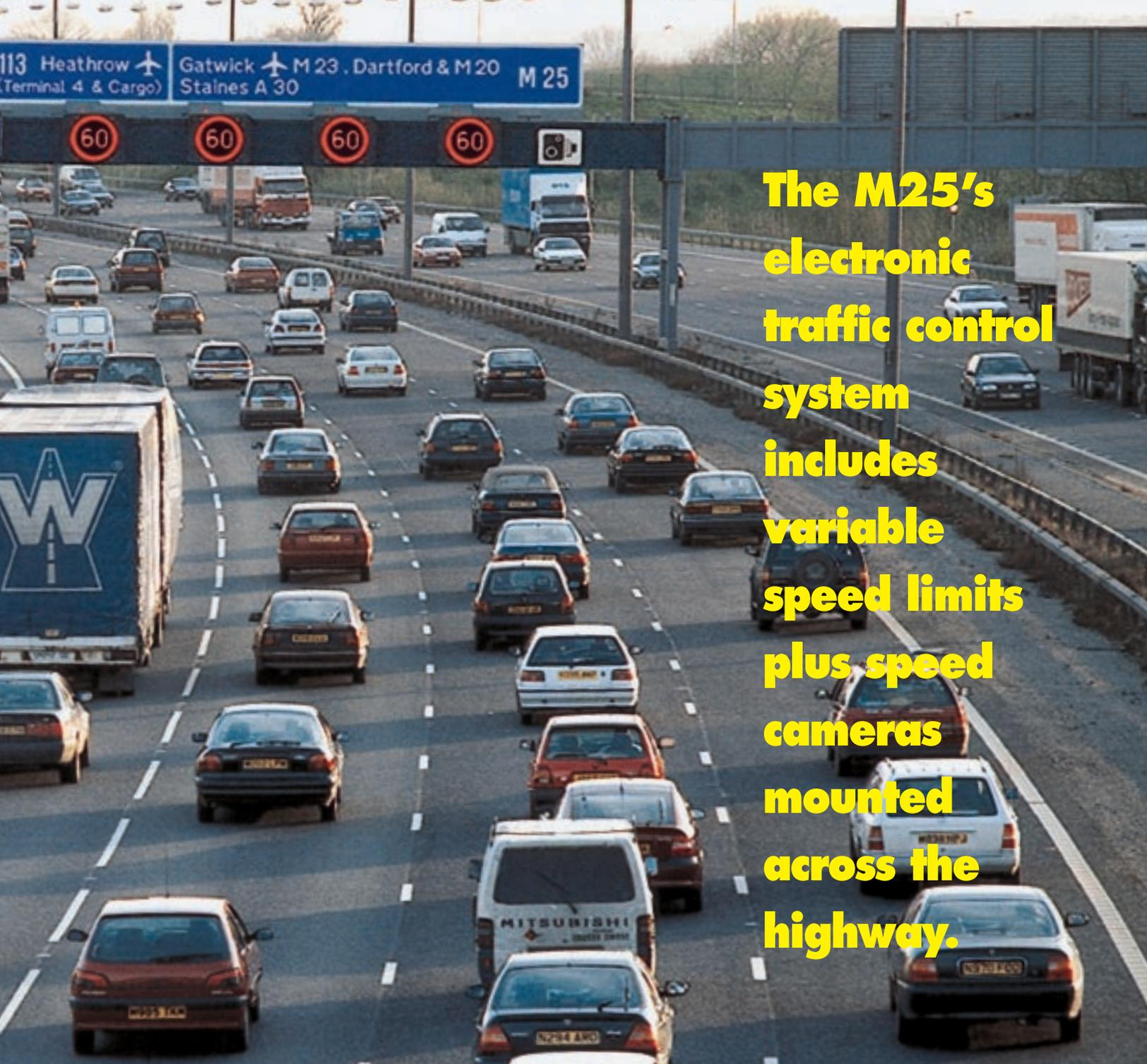
**The M25's electronic traffic control system includes variable speed limits plus speed cameras mounted across the highway.**
